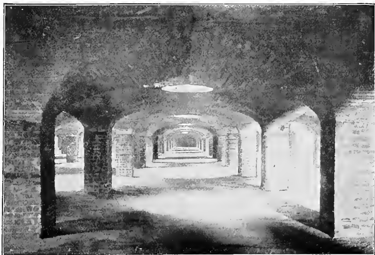
INTERIOR OF A FILTER, READY FOR USE.
